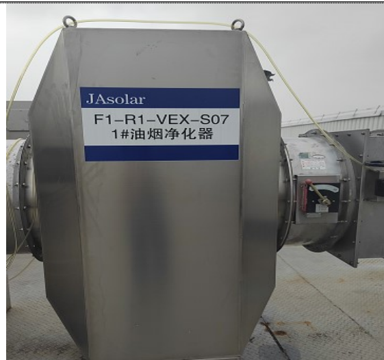
层压废气-静电除油
