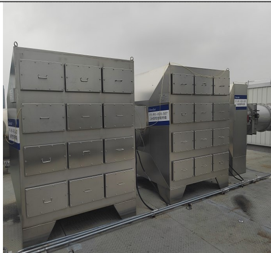
层压废气-静电除油+二级活性炭吸附
