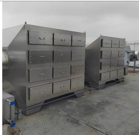
接线盒焊接、固化废气-干式过滤+二级活性炭吸附
